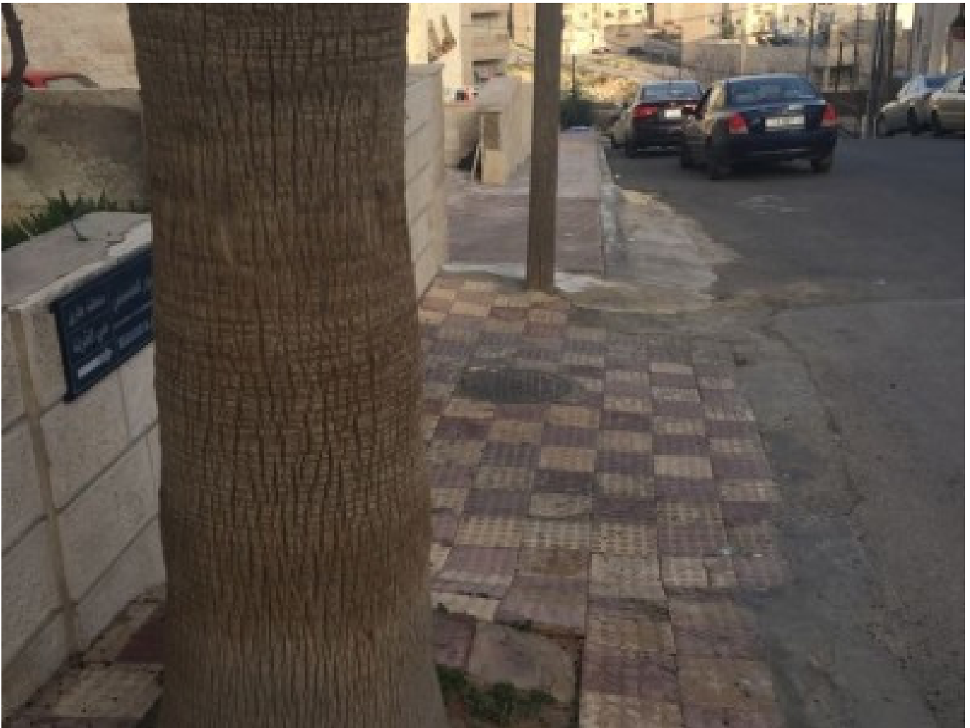
Fig. 1: Amman Sidewalk Quality, North Station Area. Photo by Muna Bata
