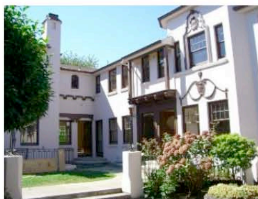
Fig. 7. Stucco finish, wooden doors and windows
