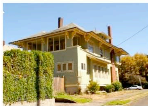
Fig. 9. Roof details– wide eaves and knee braces
