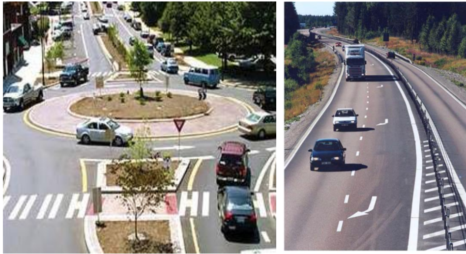
Figure 6 Roundabout (on left) and a 2+1 road with a center barrier (on right) (Source: Derr. 2003, 13)
