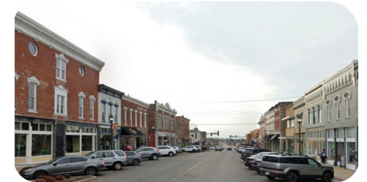
E Walnut Street looking West towards N 2nd
