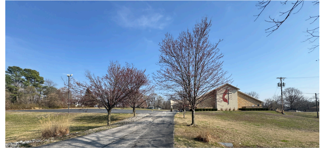
Looking east from Highway 112 towards Elm Springs United Methodist Church
