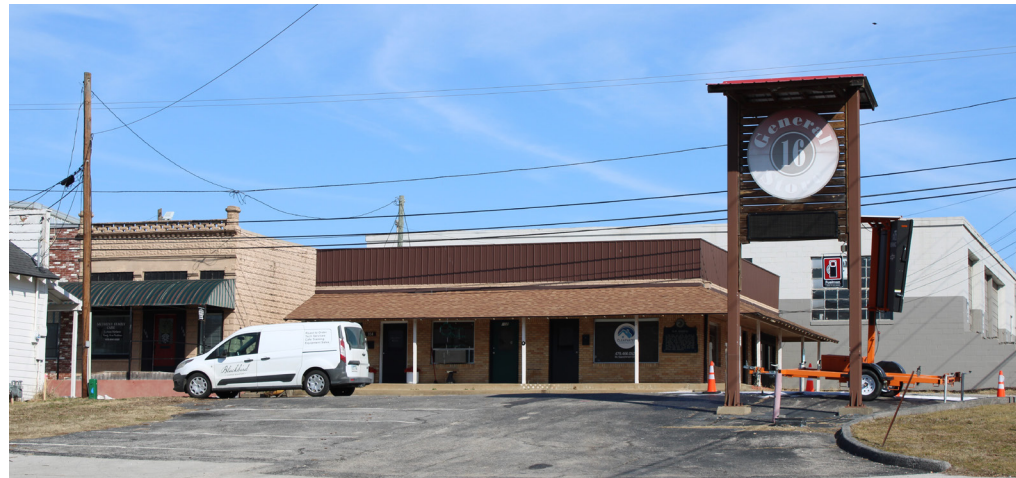
Looking northwest from Highway 112 south of Water Ave
