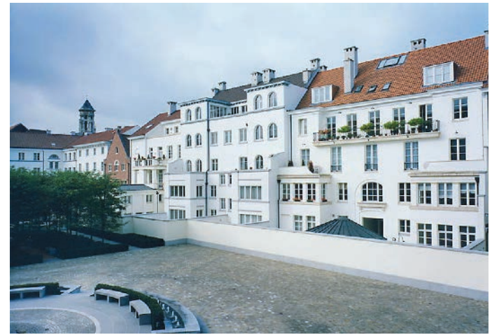
The residential row as seen from the central courtyard. Photo courtesy Fortis A.G.
