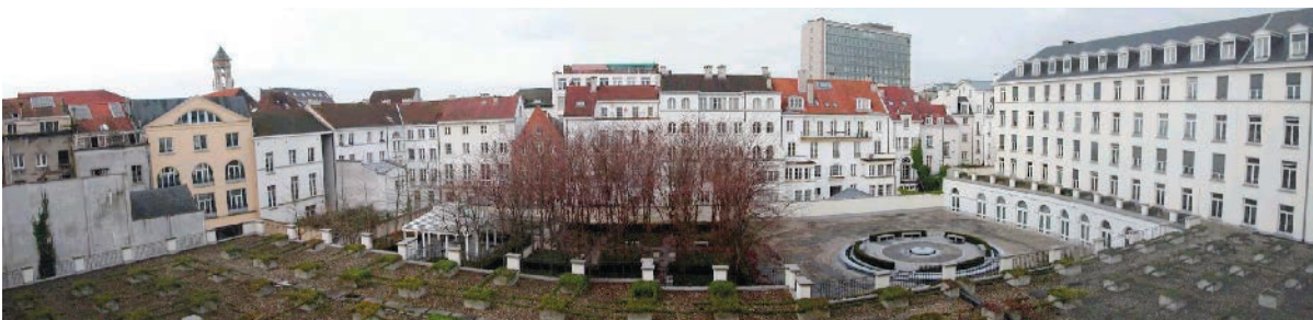
Above: Panorama of site before construction. Below: Panorama from the same vantage point after construction is completed. Photos courtesy Fortis A.G.
