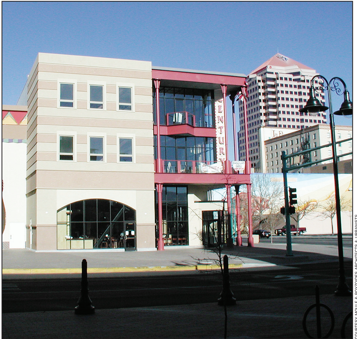
The Century Theaters block serves as the cornerstone of downtown Albuquerque’s revitalization effort.
