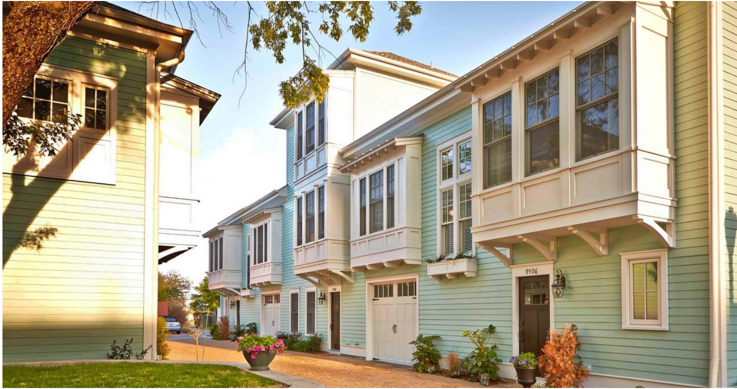
Liner buildings used to screen the view of parking lots
