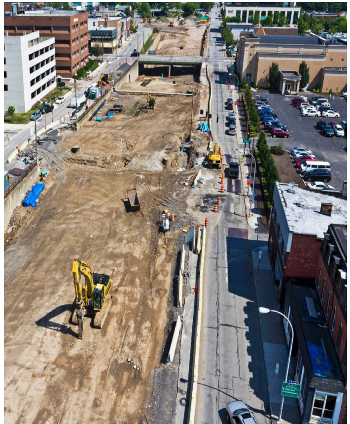
Rochester, NY began in 2017 to fill in its Inner Loop and restore the city’s urban fabric.
