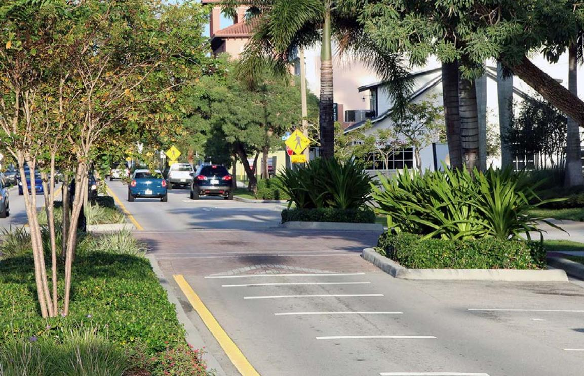
*On US 1 in Stuart, Florida, the desired target speed is achieved by using a combination of tools—a raised crossing, curb extensions, inset parking, trees and ground cover—all used to slow traffic as the road approaches a key intersection to enter the quaint downtown.*
