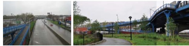
174th St Pedestrian Bridge Entrance
