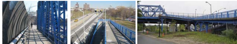
174th St Pedestrian Bridge Entrance
